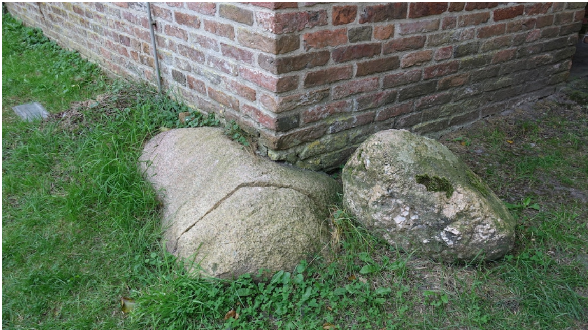
An early instance of deliberate integrality: glacial boulders are integrated into the foundation of the 12th century St Magnus church in Anloo, province of Drenthe, the Netherlands. The area is known for its neolithic dolmens, constructed from glacial boulders like these (photo Emily C. Thomas 2024).
